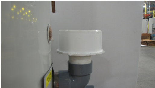
Step 3: 4" to 6" Bushing/Reducer Installed
