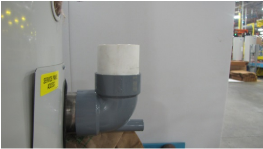
Step 1: Condensate Elbow with Small Length of 3" Pipe Installed
