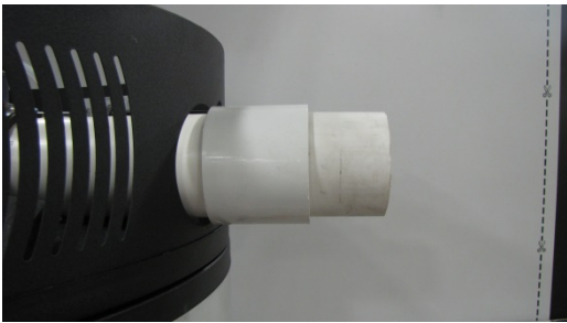
Step 1: Coupling with Small Length of 3" Pipe Installed
