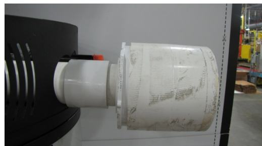
Step 4: 6" Pipe Installed
