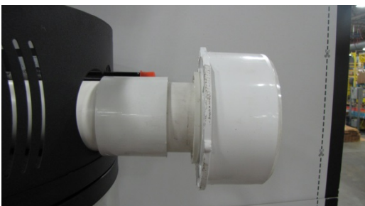
Step 3: 4" to 6" Bushing/Reducer Installed
