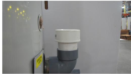
Step 2: 3" to 4" Bushing/Reducer Installed
