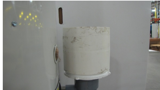
Step 4: 6" Pipe Installed
